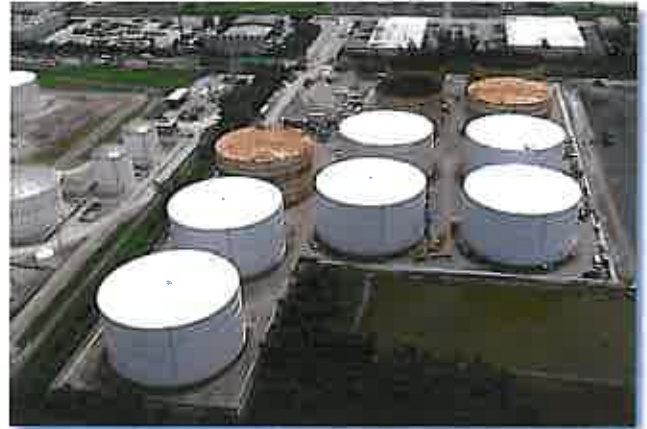
Prior to construction of these 11 fuel storage tanks, underlying soft clayey silt with peat lenses was improved by mass dry soil mixing to control settlement.
